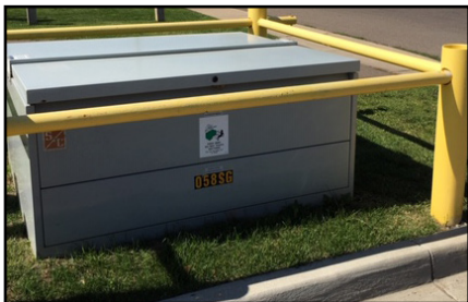
Padmount Switchgear
