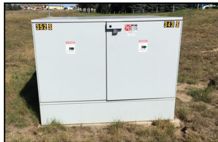
Padmount Switchgear
